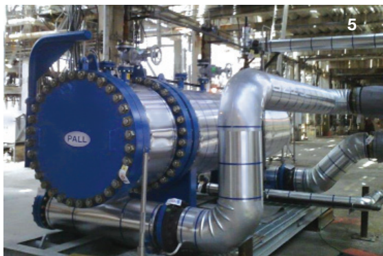
1) SepraSol™ Plus Coalescer: compressor protection; 2) AquaSep® XS Coalescer: steam stripped diesel; 3) Filter Rental Fleet: quick problem resolution; 4) AquaSep XS Element: reliable diesel deahazing; 5) Ultipleat® High Flow Filter: catalyst guard
